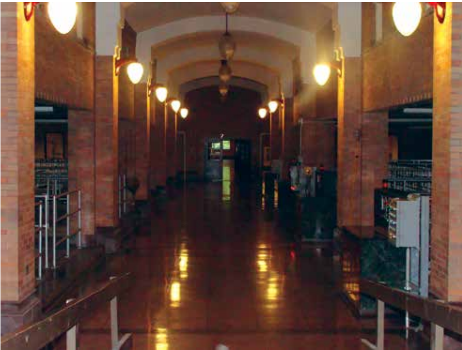
Figure 2. Main filter gallery at a well-maintained Lake Erie drinking water treatment facility. Although some of the instrumentation panels are of modern design, the plant itself was constructed in 1940.
