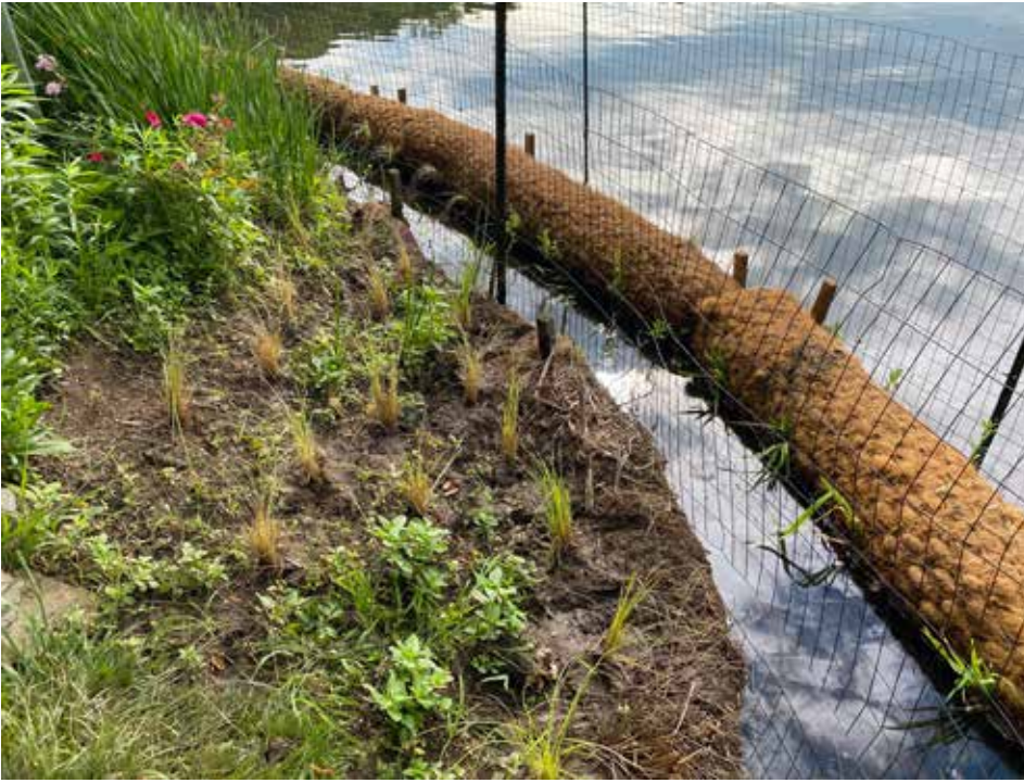
Figure 4. Established coir logs along shoreline of Reston area lakes.
