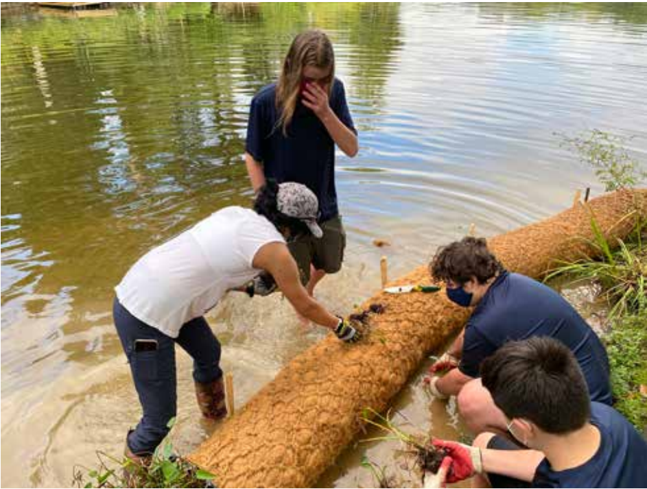
Figure 5. Installation of coir logs.
