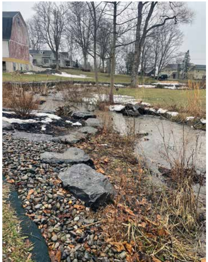
Figure 3. Stabilization efforts along lower Willow Creek during storm capturing sediment.
