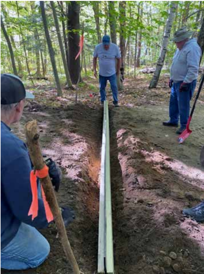
Figure 6. Lake resident installing a razor for runoff control.
