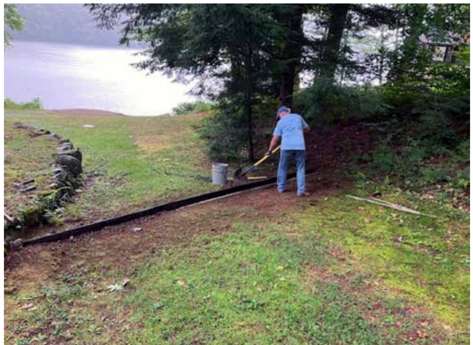
Figure 5. Lake resident installing a razor for runoff control.
