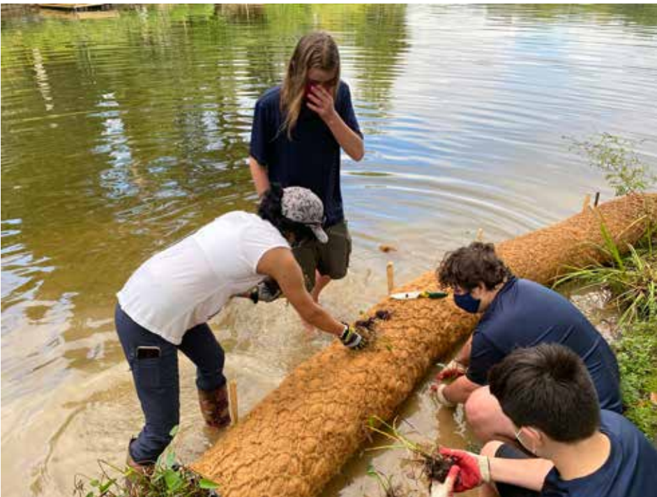
Figure 5. Installation of coir logs.
