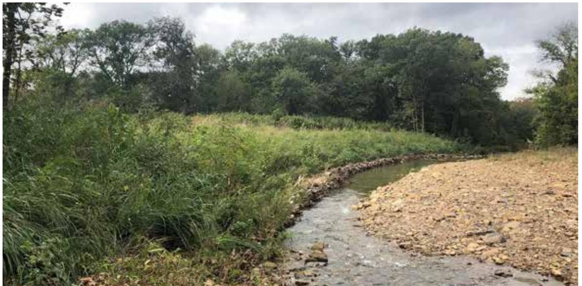
*Figure 2. West Fork White River Watershed Initiatives: restored streambank on Rock Creek using EQUIP funding. Upper photo is site prior to restoration showing eroding cut-bank; middle photo shows restored streambank with toe-wood structure and revegetated constructed soil lifts; bottom photo shows revegetated terraces planted with native trees, shrubs, and grasses and seeded with native grasses and wildflowers.*
