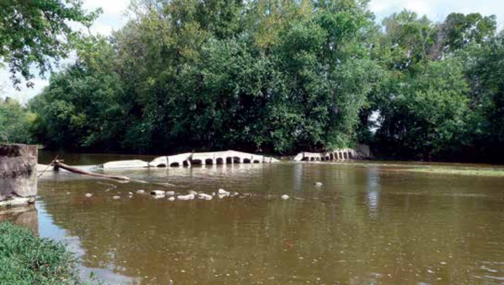
Figure 4a. Mexico Dam before removal.
