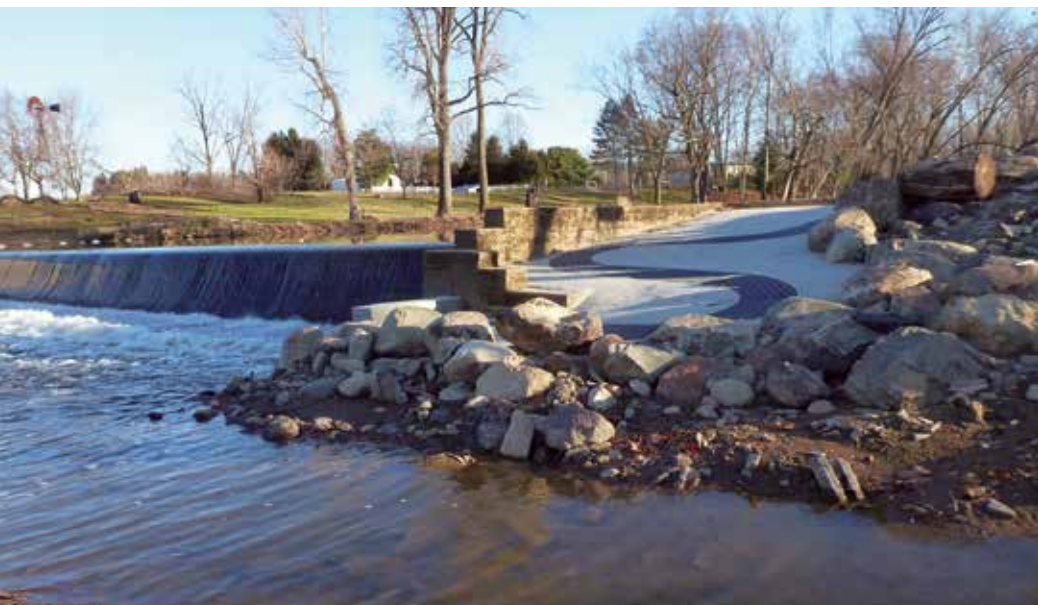
Figure 5. Fish ladder at Stockdale Mill Dam.
