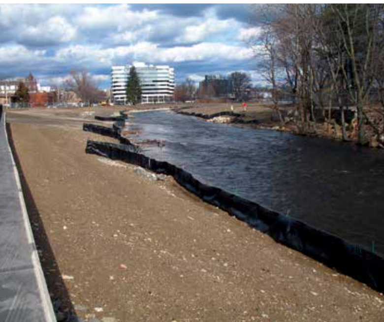
Figure 5. Mill River Stamford, CT, immediately following dam removal.
