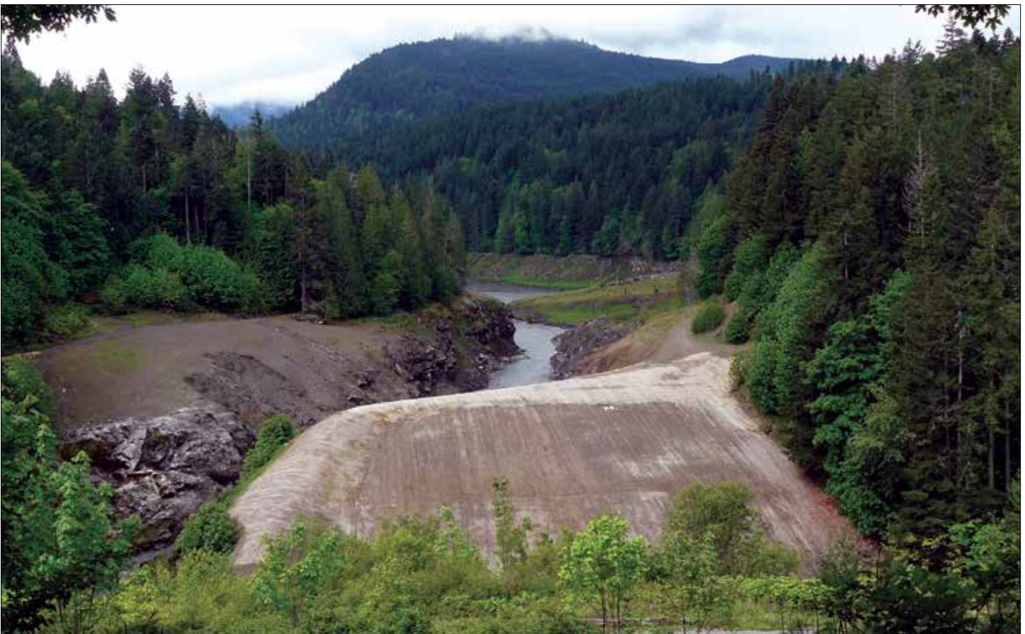
Figure 5. After removal of Elwha Dam with river back in its original channel. Source: Creative Commons. Photo by Zandcee.
