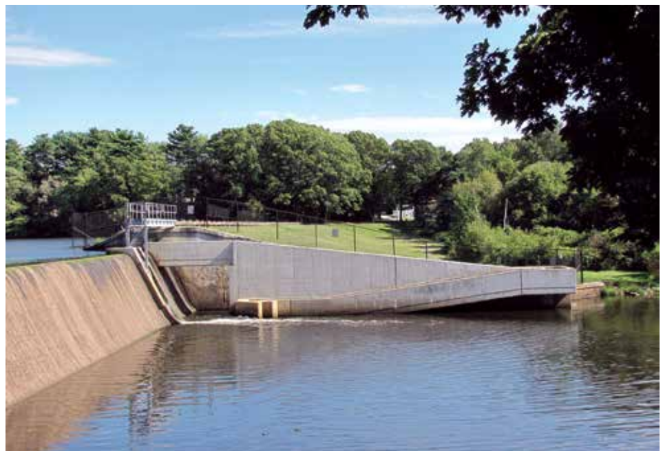
Figure 3. Fish ladder on the Hunts Mill Dam in East Providence, Rhode Island. The fish ladder entrance is in the top left of the photo.
