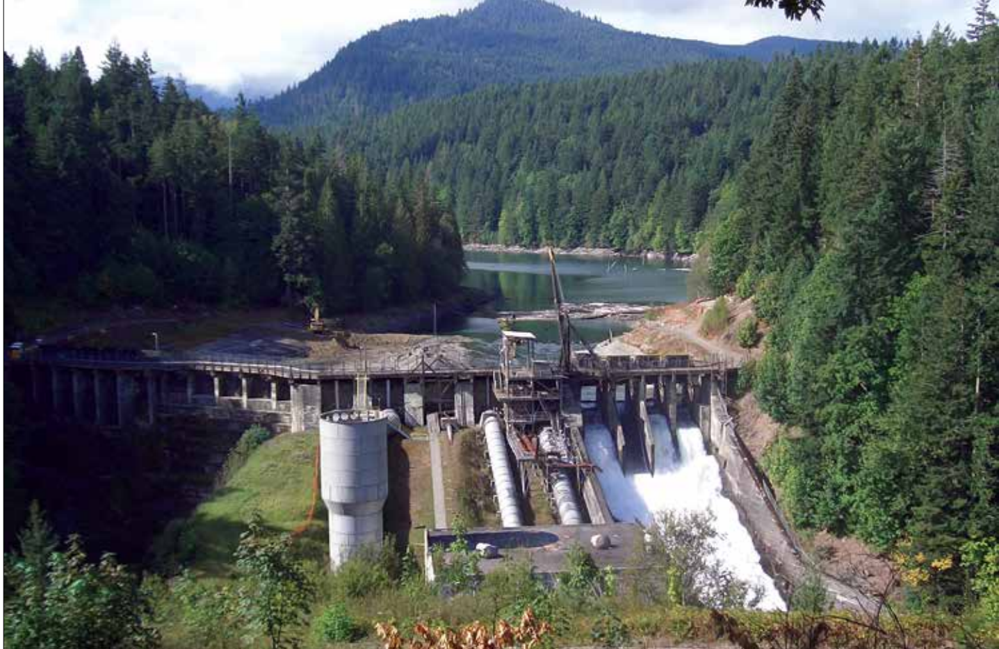
Figure 4. Elwha Dam early in the deconstruction process. Water has been diverted to the spillway on the right to lower the Lake Aldwell. Source: Creative Commons. Photo by Ben Cody.
