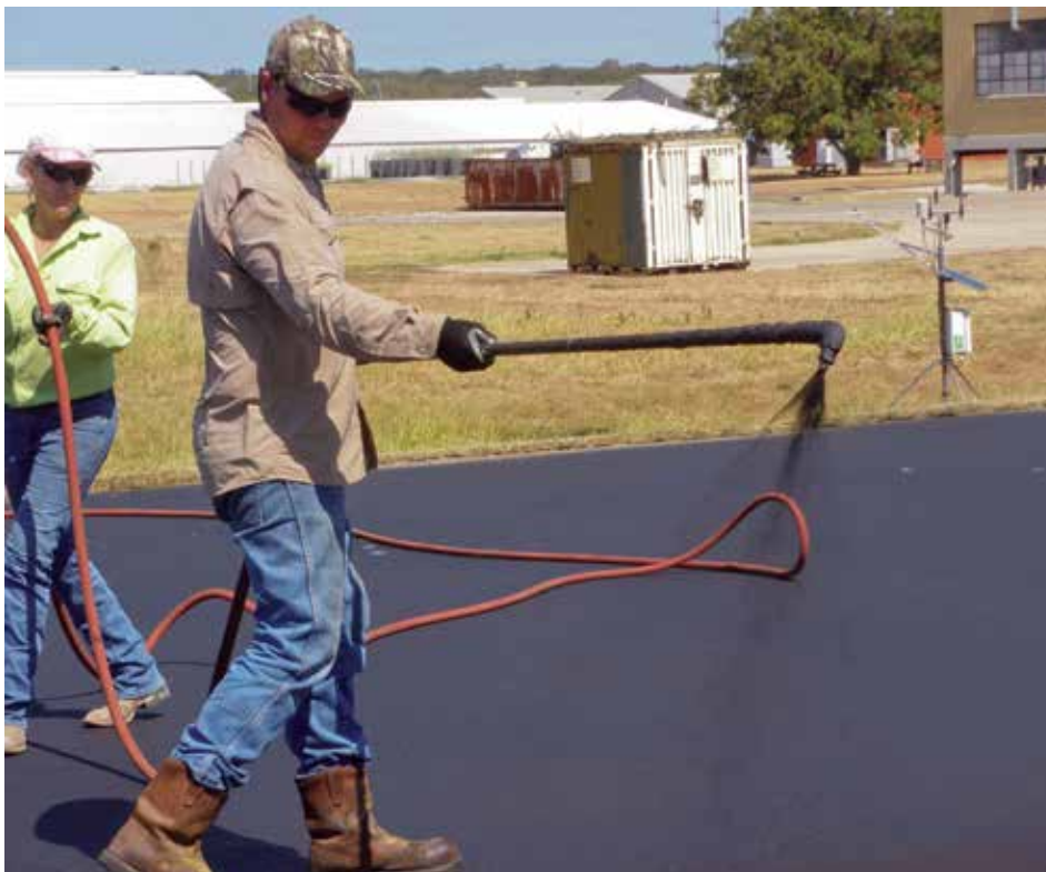
Figure 3. Individuals can be exposed to several lower molecular weight PAHs in coal-tar-based sealcoat that are volatile and emanate from asphalt surfaces after sealcoat is applied. Risks associated with exposures to these compounds has yet to be studied, though any such contact would be expected to be greatest for professional applicators of sealcoat products and relatively low for others. Photo: Peter Van Metre.
