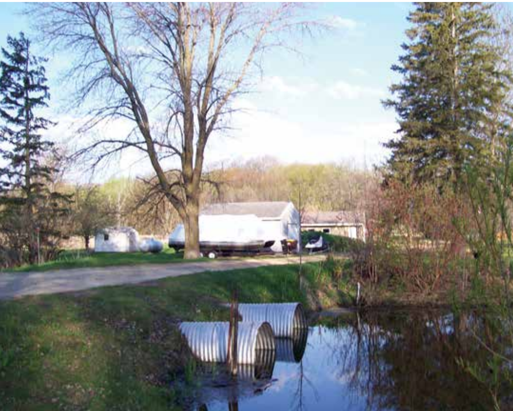
Figure 4. The outlet culverts were replaced to further help prevent shoreline erosion due to high water.
